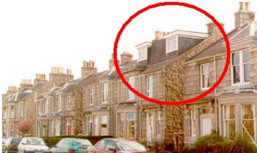
Example of a poorly designed roof extension – Dormers are too large, dominating the roof slope, and use of substantial infill panels and slated aprons contributes to bulky appearance
